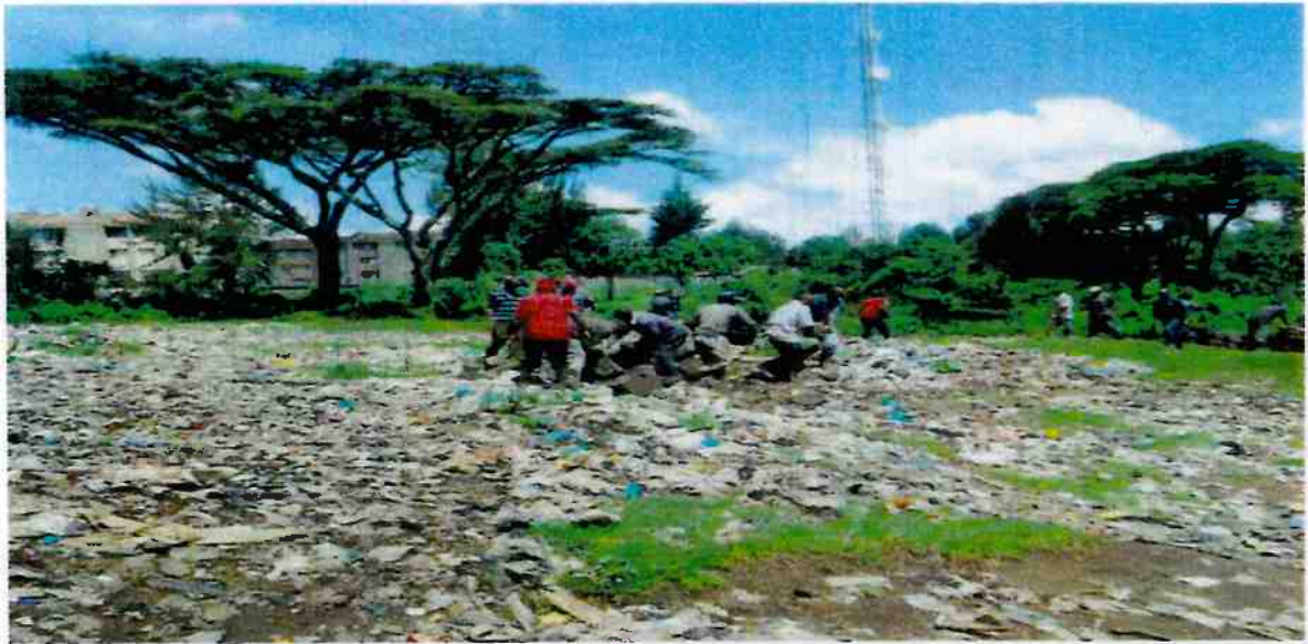
A section along the River Njoro undergoing rehabilitation
